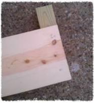
BOARD TO POST USING TWO NAILS EACH
